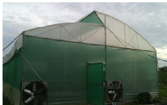
Fig. 1: High-tech poly green house structure
